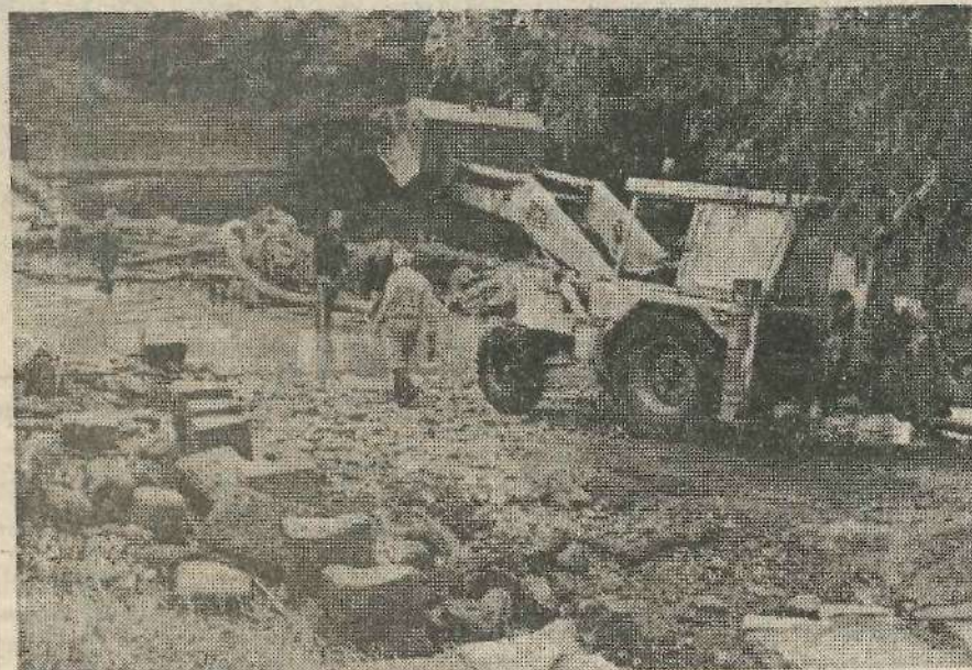
The stepping stones across the River Wharfe at Ben Rhydding were repaired in June, after having been in a state of disrepair for over ten years since about a dozen were washed away in a severe storm. Picture by Richard Beckwith, Ilkley.
