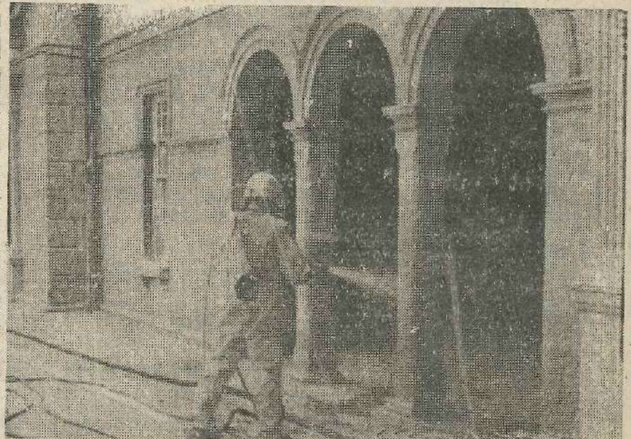
Work started in October on a major clean-up scheme at Ilkley Railway Station, beginning with sandblasting of the building, which dates back to the 1860's.
