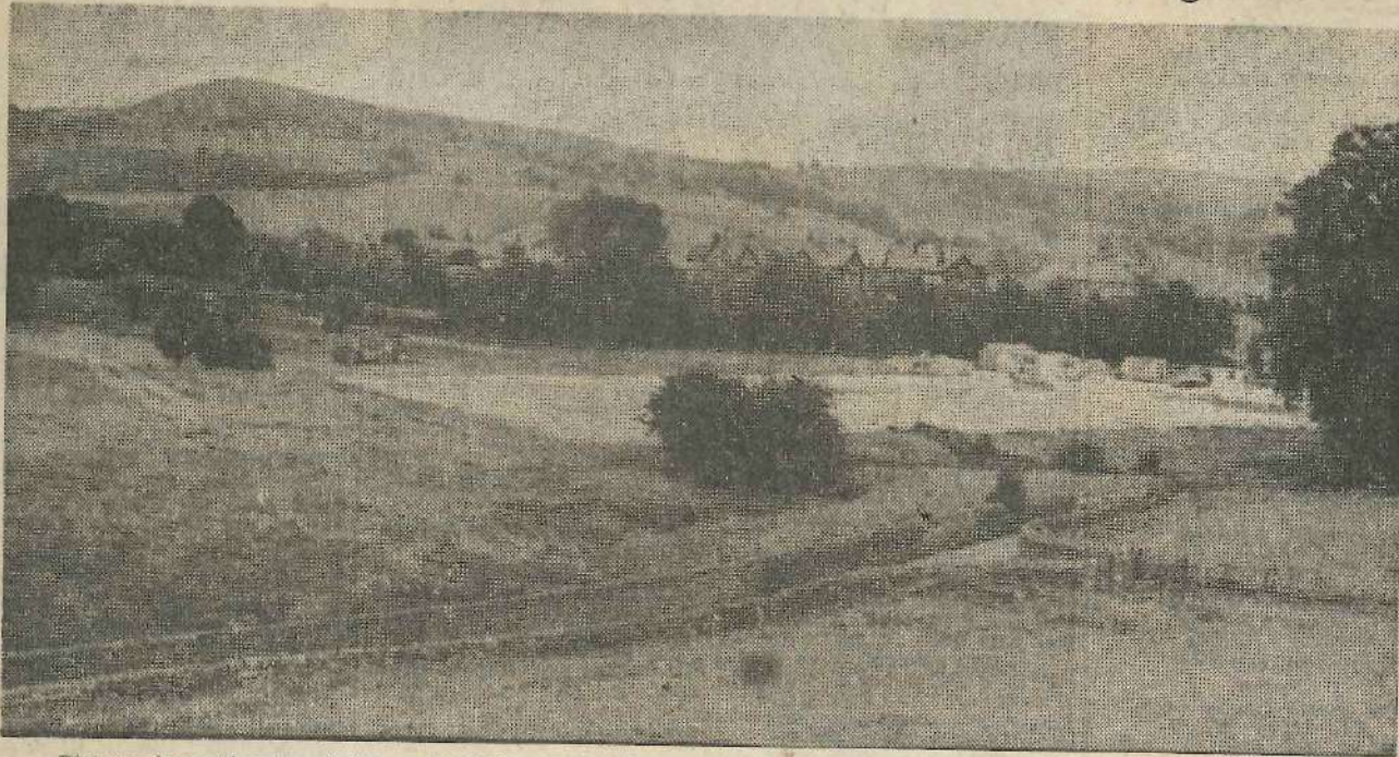
Picture shows the site of the new middle school being built at Addingham, with Back Beck Lane in the foreground and Beamsley Beacon in the distance.
