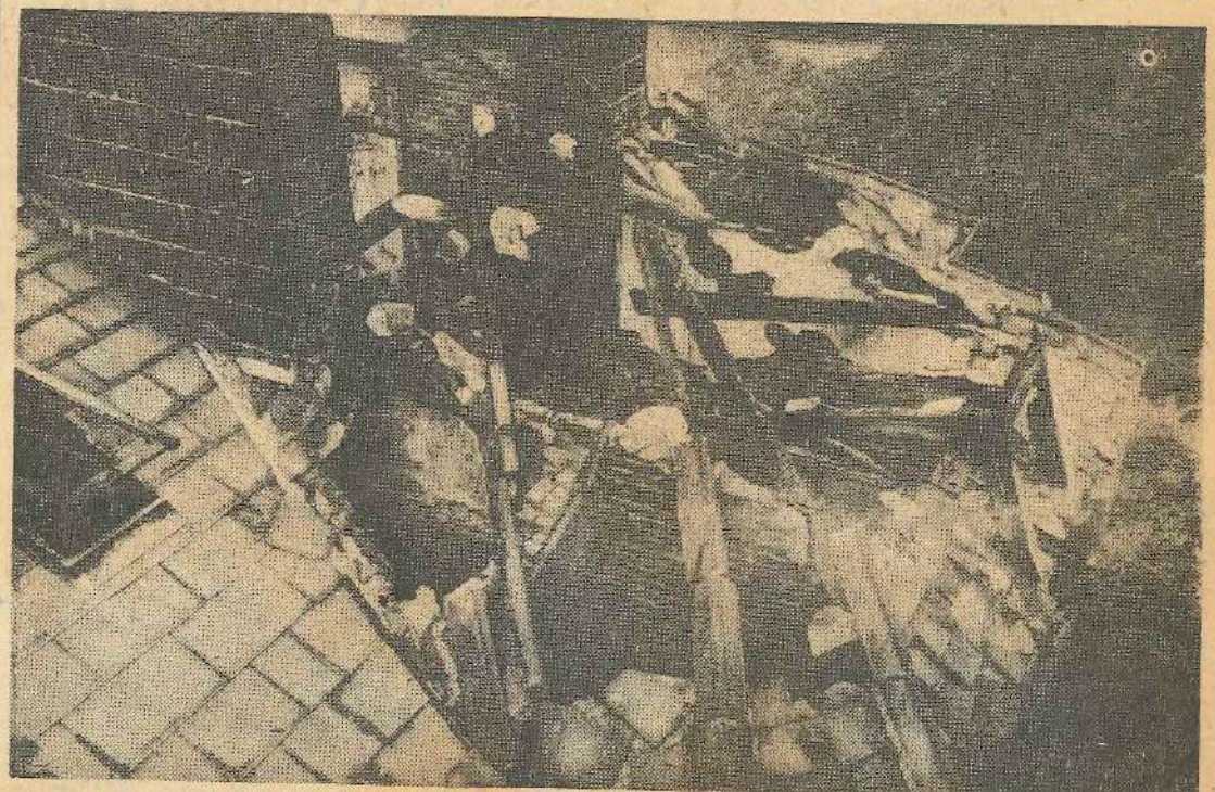
A picture from the roof looking down into the lift shaft of the Ilkley Moor Hotel. It was after the fire had reached this section that it spread rapidly to other parts of the hotel.
