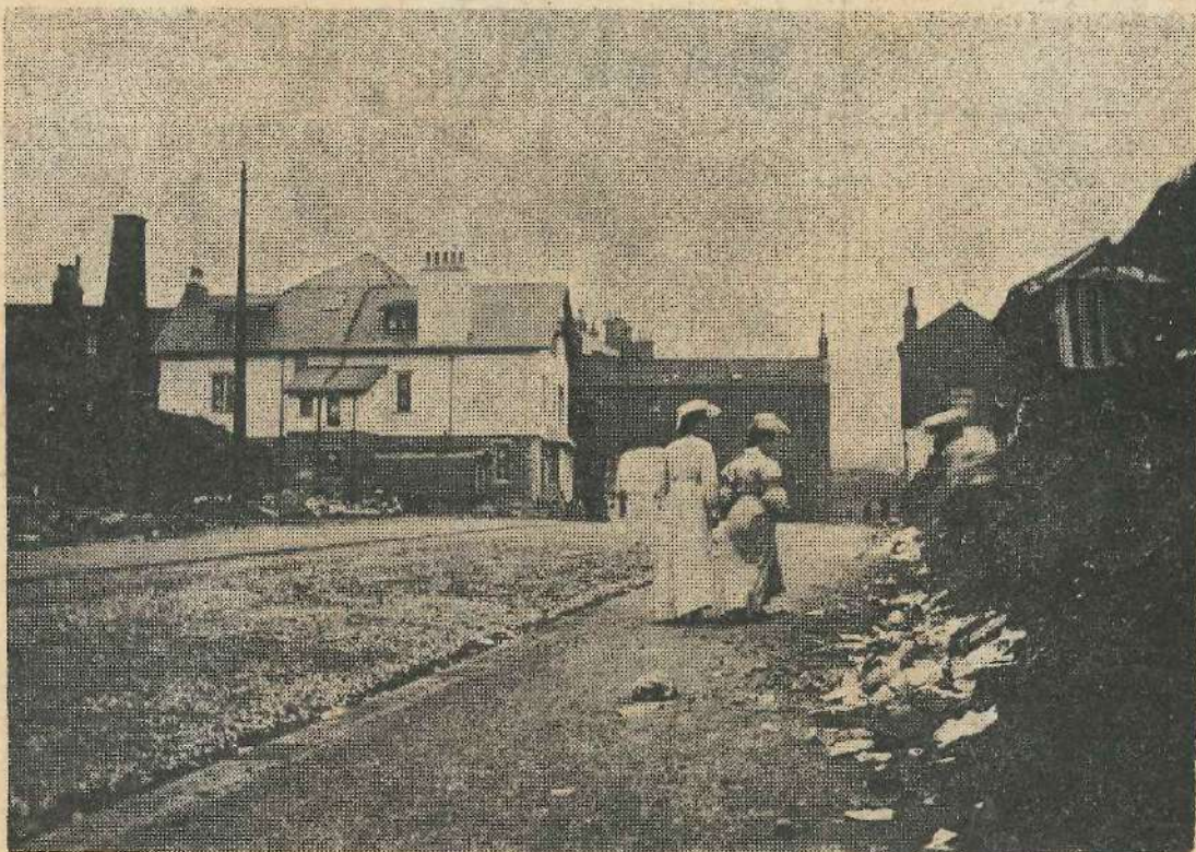
This picture was taken about the time the old Wheat Sheaf and the Star which provide a background for the two women in the picture which stood together at the bottom of Brook Street were demolished. The white building on the left is the new Star, the chimney is part of the old gas work. The gable end to the right is that of the Wheat Sheaf and it will be seen that New Brook Street is in the making.
