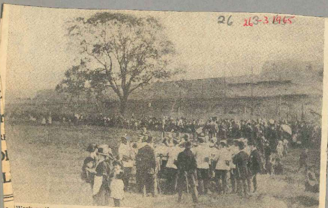
Work on the railway wall on the down platform from Skipton was still in progress when this picture was taken from the old cricket field on which Trafalgar Road, Victory Road and Nile Road were built.
