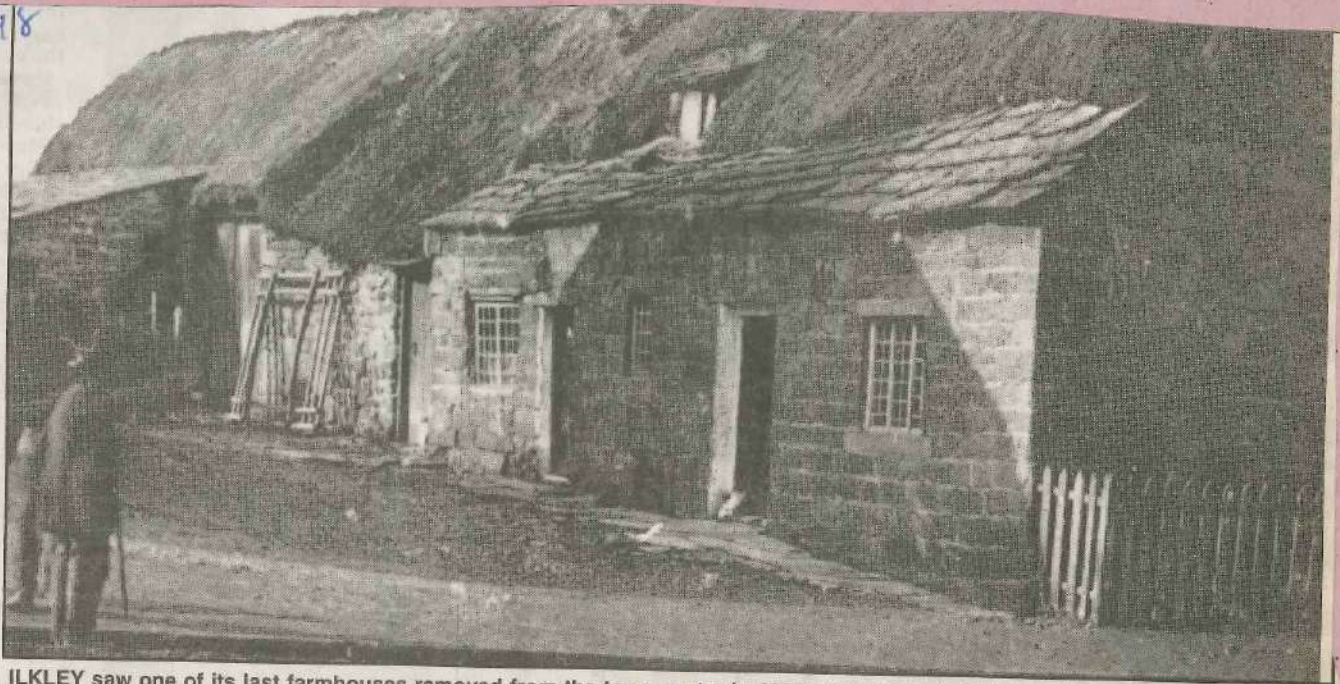
ILKLEY saw one of its last farmhouses removed from the town centre in 1868 when these buildings (pictured) were demolished to make way for Gothic House (now occupied by Boots the chemist) and for a new street to be known as Hawksworth Street. The farm was owned by Billy Hawksworth and was purchased by John Shuttleworth (founder of the Ilkley Gazette) who built Gothic House on the site.
