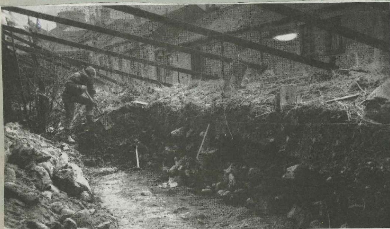
EVIDENCE of the establishment of the Roman Fort of Olicana at Ilkley in AD 97 and of its development through to the fourth century was unearthed during the course of excavations in 1962. The picture shows a portion excavated immediately behind the poster hoardings which flanked New Brook Street. The stones were of little significance but in the floor of the trench were post holes connected with an early wooden building. Brian Hartley, of Leeds University, who was in charge of the excavations, said one of the most interesting discoveries had been the traces of late second century timber buildings behind these poster hoardings. There was evidence they had been destroyed during a native revolt at the end of the second century. The buildings in the background are those of the stables and outbuildings of the Wheatshaf Hotel which were later demolished.
