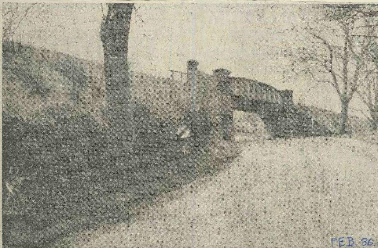
Scenes from the past this week takes a look at the A65 trunk road in Skipton Road near Hollin Hall Farm looking west towards Addingham. The closure of the railway from Ilkley to Skipton and the Dales in the 1960s gave road engineers the opportunity to improve the road at this point by removing two bends, one of which now serves as a lay-by beyond where the bridge carried the railway across the A65.
