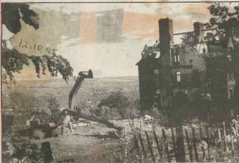
The last remnants of Semon Home are demolished
