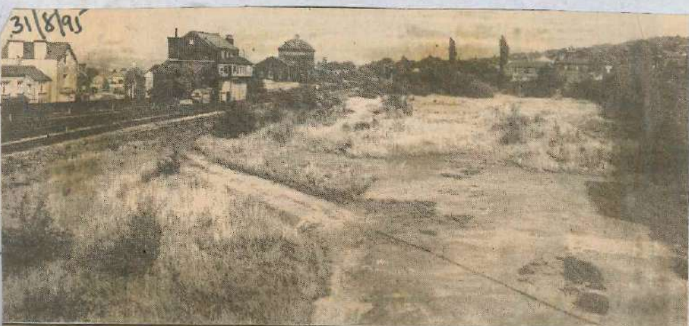
LAND in Springs Lane which served for many years as Ilkley's railway goods yard was transformed in 1983 when it was redeveloped for a new Hillards superstore which, in 1987, was taken over by Tesco.
