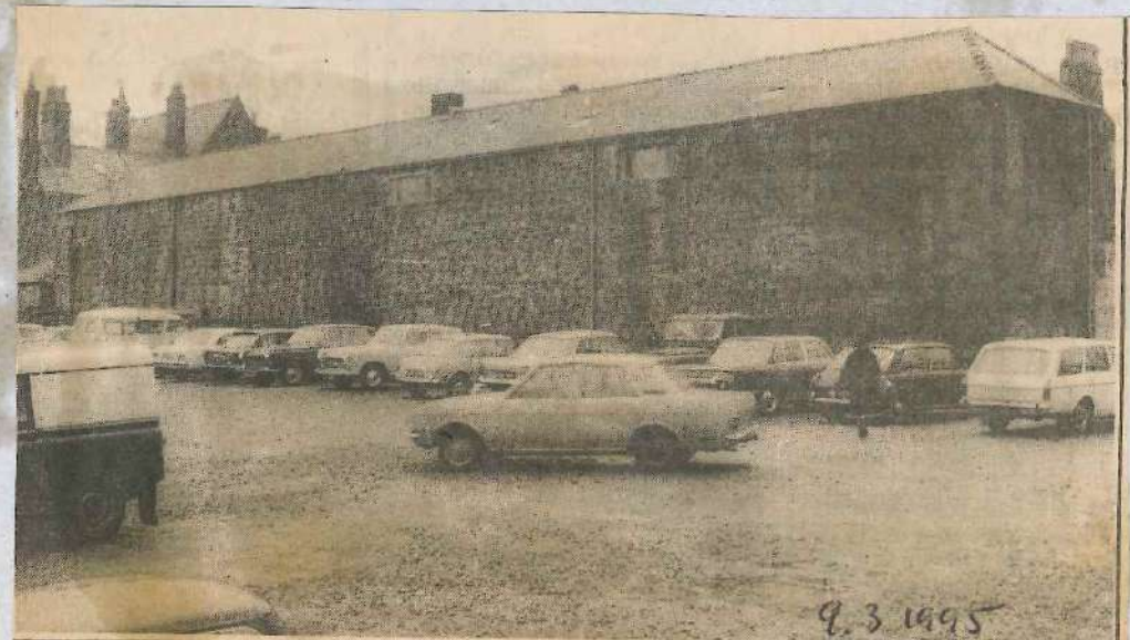
A row of shops to become what is now known as the Grove Promenade was formed from this warehouse which once served shops in The Grove. The area on which these cars are parked had previously been occupied by a high embankment which carried the railway west of Ilkley.
