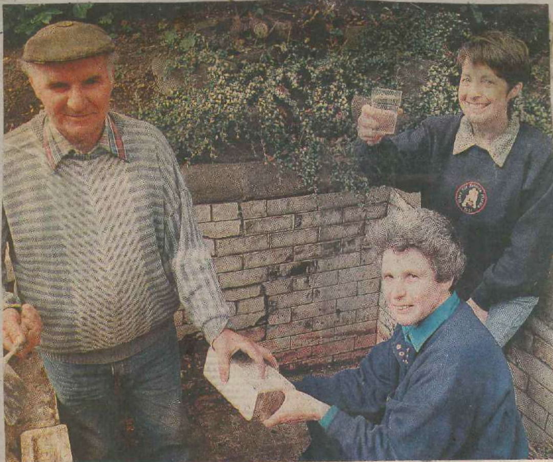
Pictured at the well are stonemason Jimmy Barker, Pat Hudson and Pat Baker, toasting the start of restoration work. Picture by Philip Bambridge, of Addingham.
