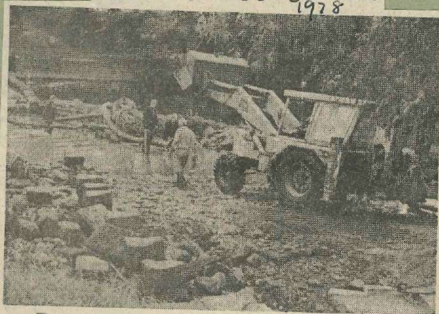
The stepping stones across the River Wharfe at Ben Rhydding were repaired in June, after having been in a state of disrepair for over ten years since about a dozen were washed away in a severe storm. Picture by Richard Beckwith, Ilkley.
