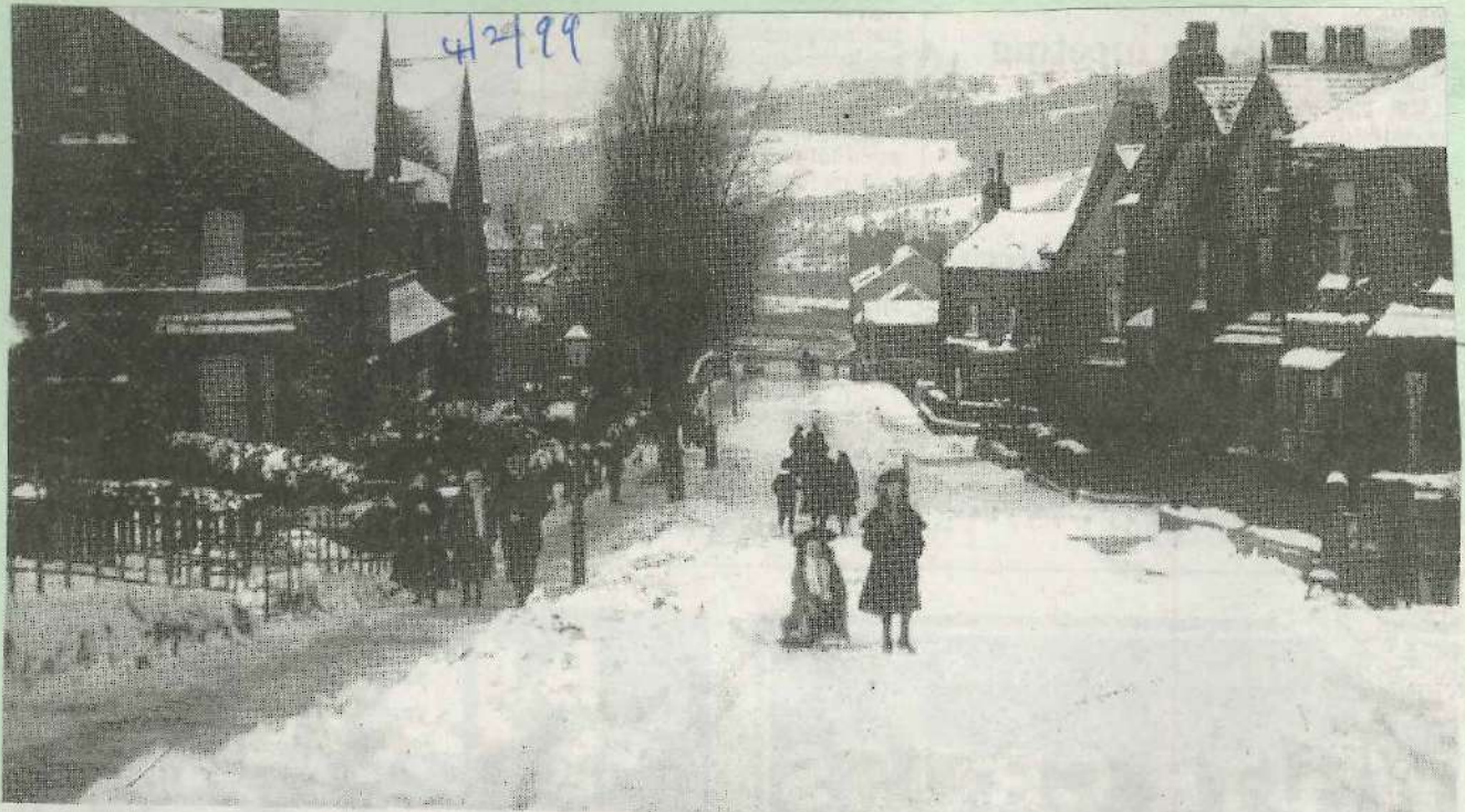
PEDESTRIANS felt free to walk in the middle of Cowpasture Road, Ilkley, to negotiate deep snow when this picture was taken in the early part of this century. It was a time when Tower Buildings stood majestically at the bottom of Cowpasture Road with its castellated tower visible in the centre of the picture. The site is now occupied by Leonfield House.
