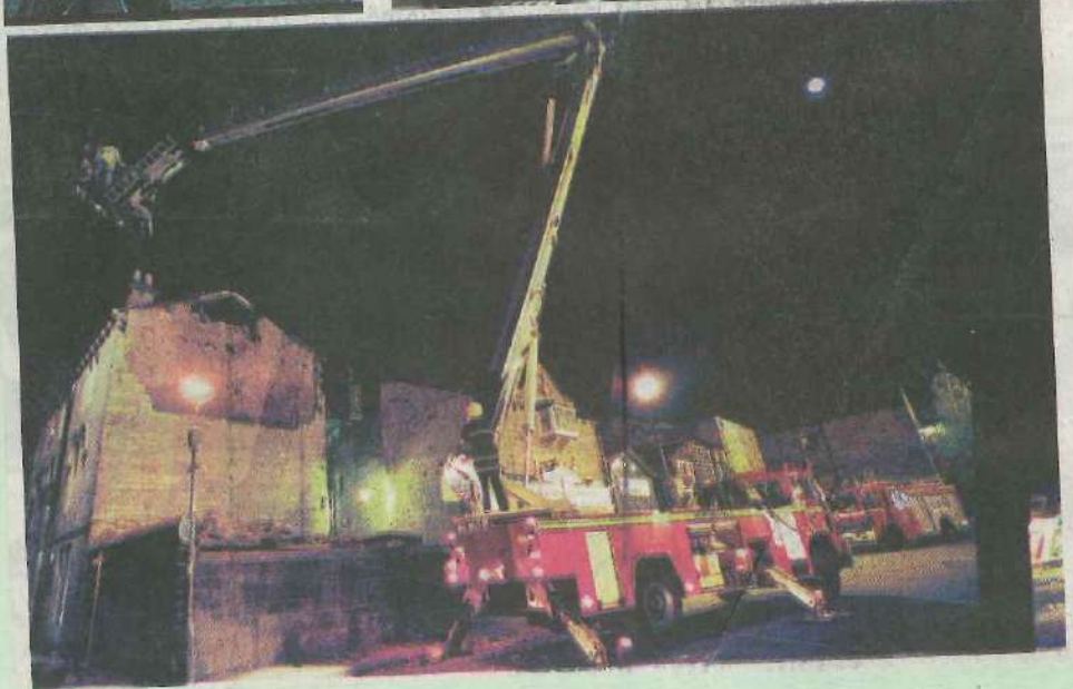
ABOVE AND LEFT: Firemen use heat-seeking equipment to check the rubble.
